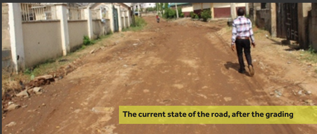
The grading of the CFHI community road
